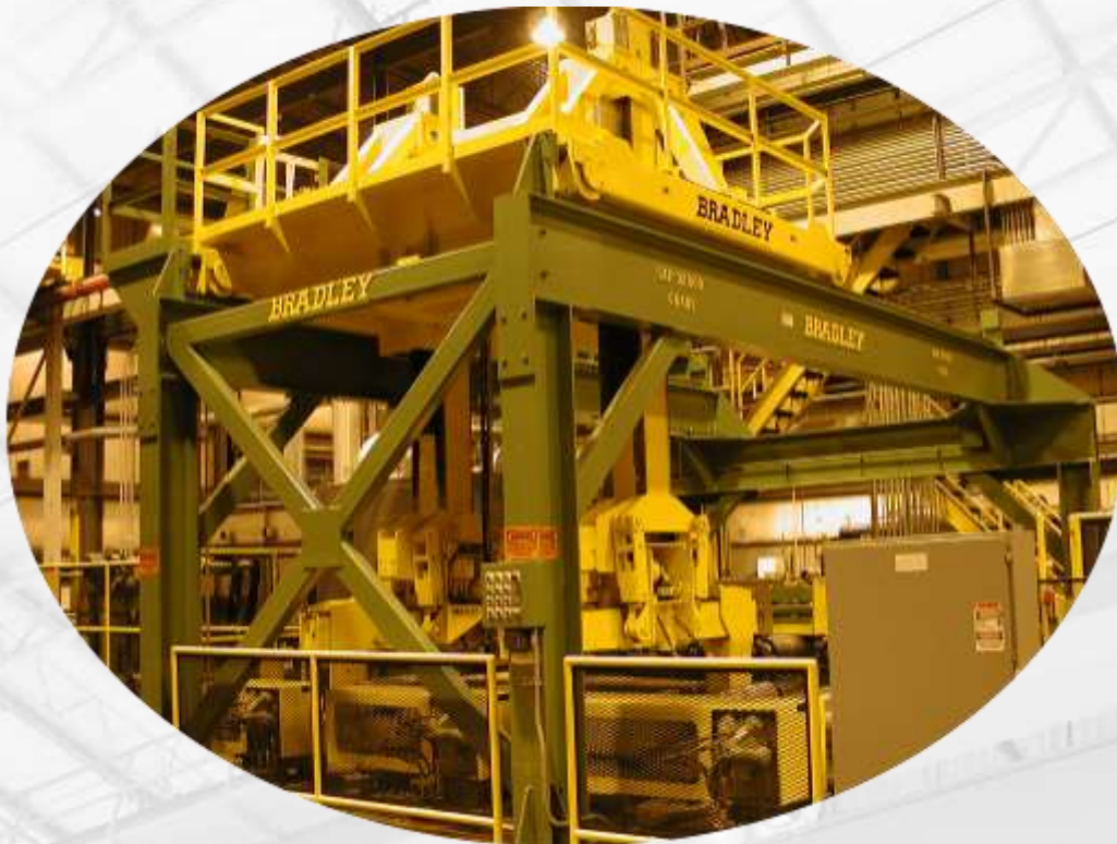
STAND-ALONE GANTRY CRANE TRANSFER STATIONS
