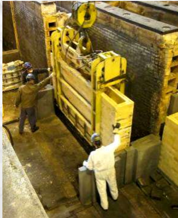
PRE-BUILT FLUE WALL BEING SET
